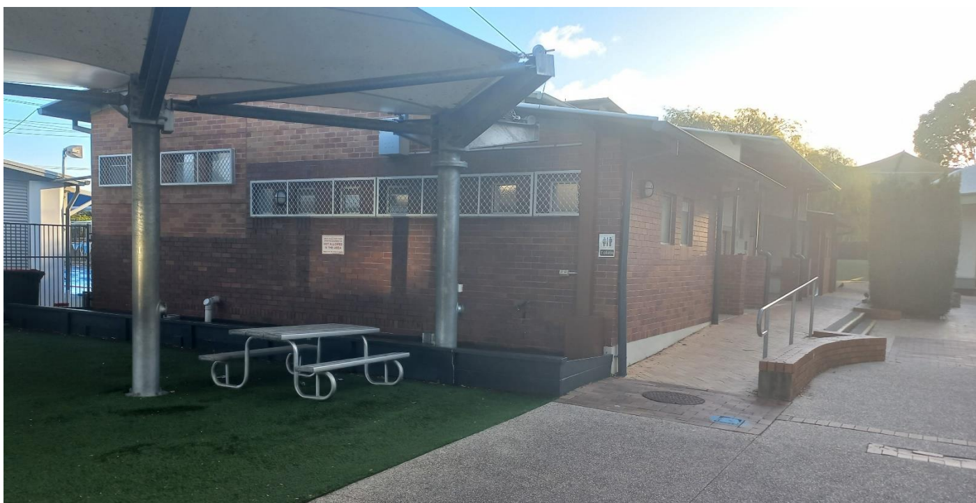
Toilet Block next to MPC
