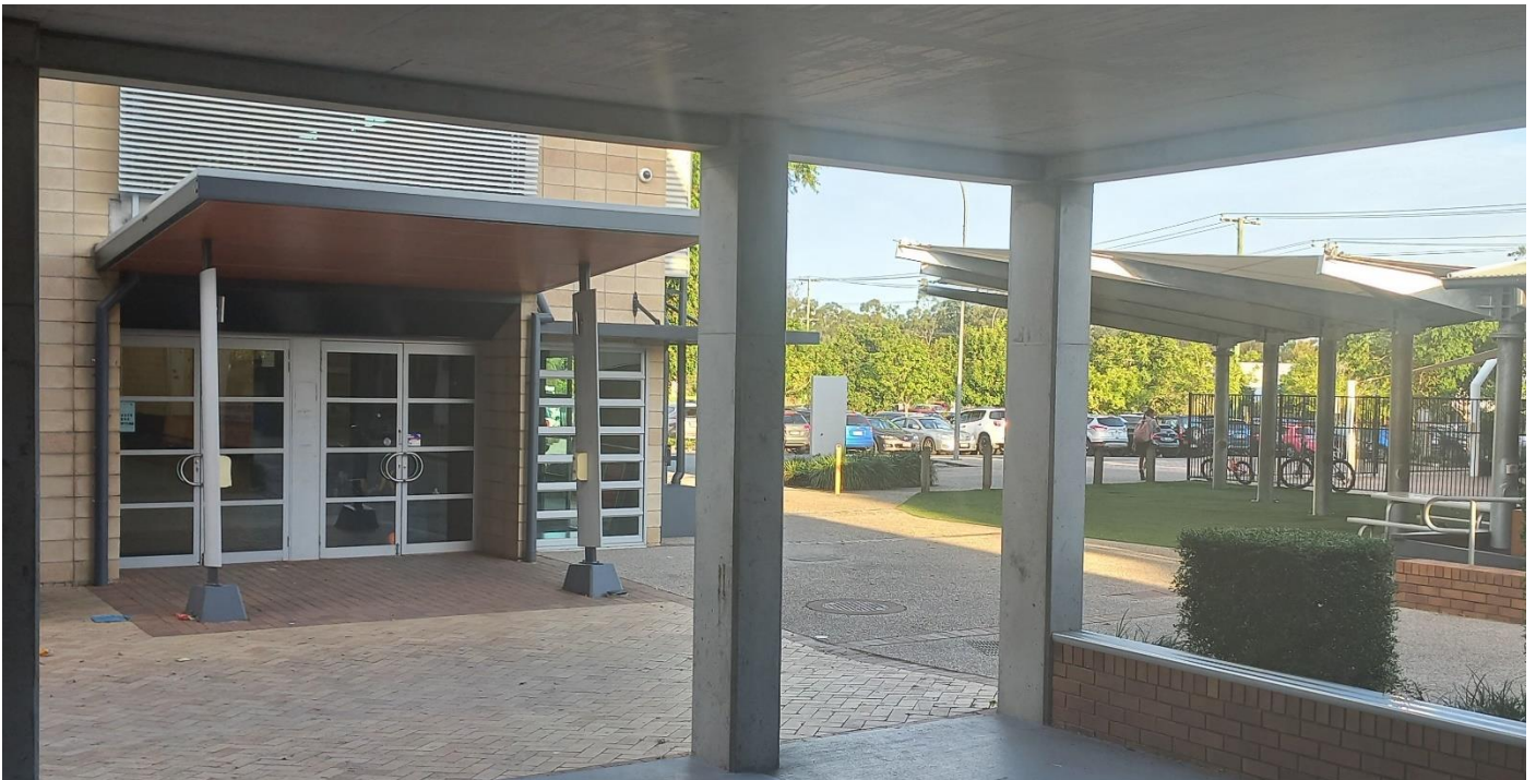
Entrance to MPC and looking towards sealed Car Park on Buchanan St
