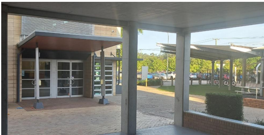
Entrance to MPC and looking towards sealed Car Park on Buchanan St
