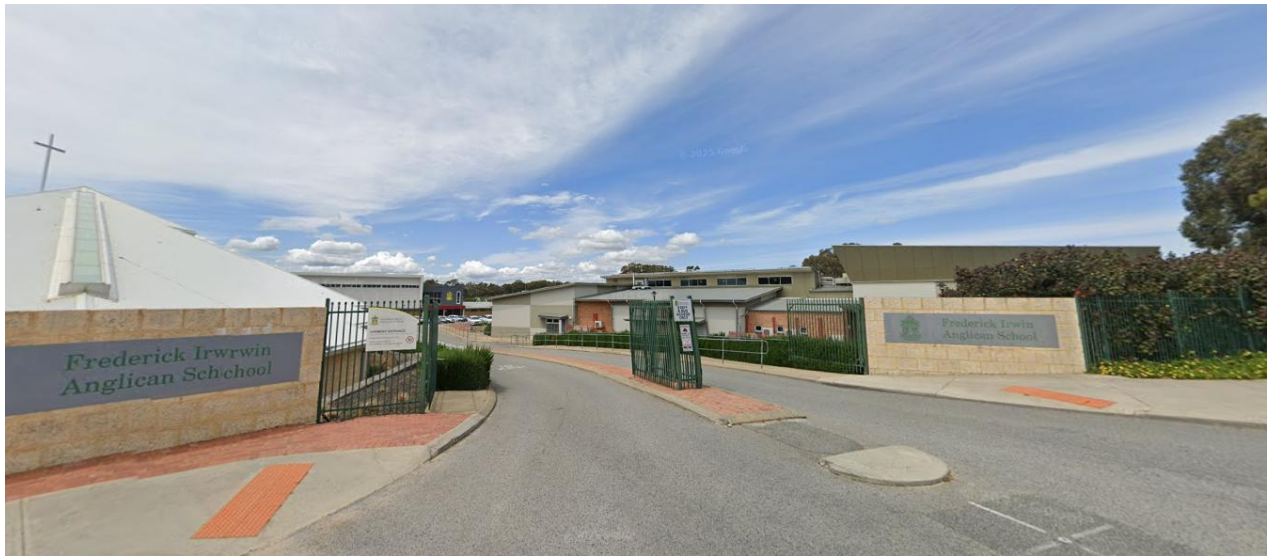
Oakmont Ave - Entrance to School
